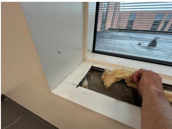
#11 Under aluminiumslysning findes isolering.
